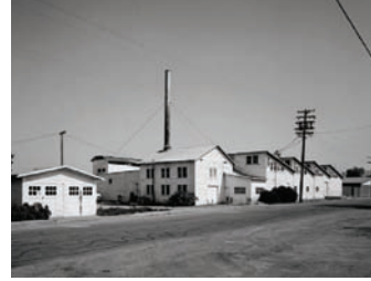
Woelffel Cannery 10120 Imperial Avenue Demolished
