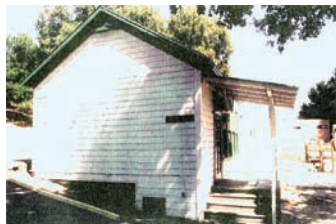
Montebello School 15101 Montebello Road
