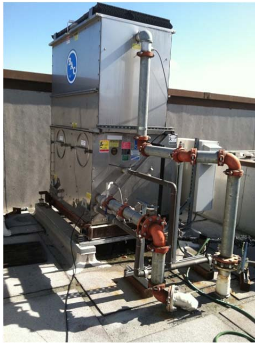
Figure 5A (Closed-Circuit 70 Ton Cooling Tower)
