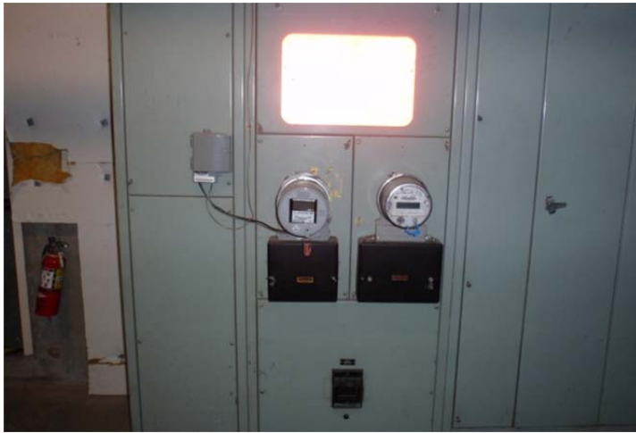
Figure 5F (Main Switchboard)
