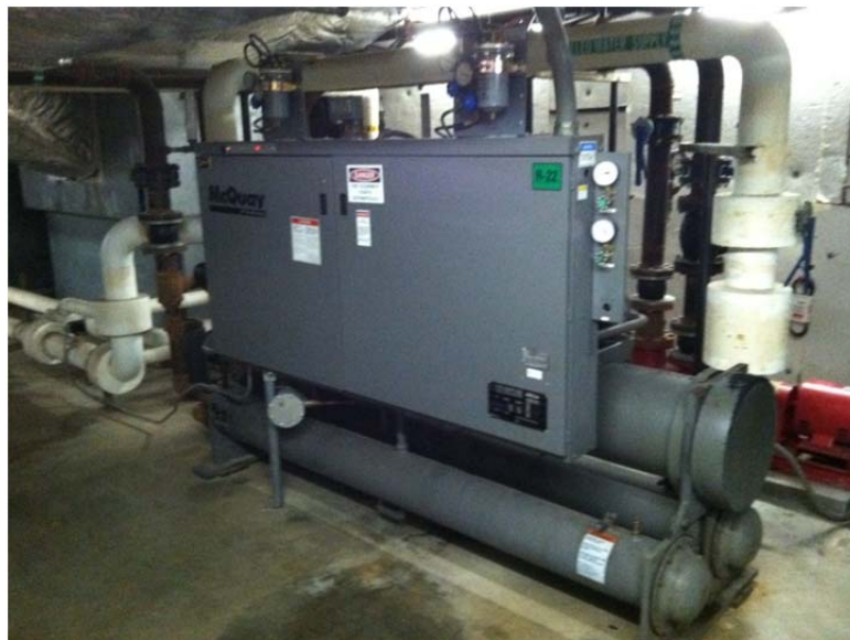
Figure 5B (Water-cooled 70 Ton Chiller)
