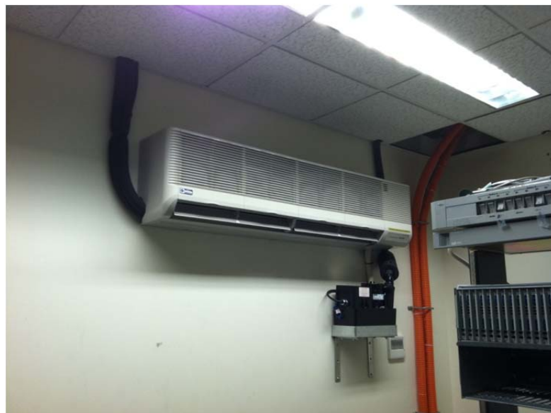
Figure 5D (Server room AC unit (1 of 2))
