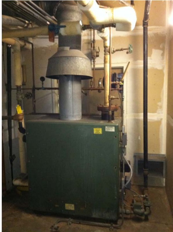
Figure 5C (Gas Fired Boiler)
