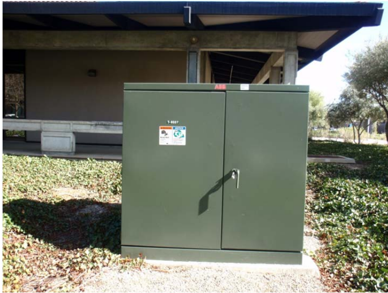
Figure 1E (PG&E Transformer)
