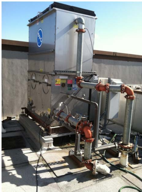
Figure 5A (Closed-Circuit 70 Ton Cooling Tower)
